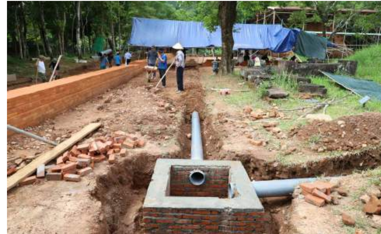
DURING: Construction of Drain Chamber at south east
