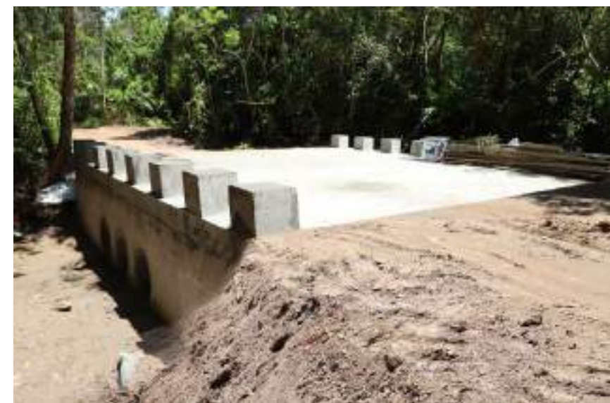
AFTER: Construction of Causeway at Cham Hut
