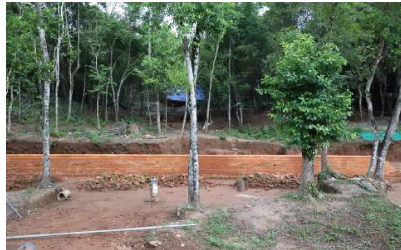
AFTER: Conservation & Restoration of East Enclosure wall
