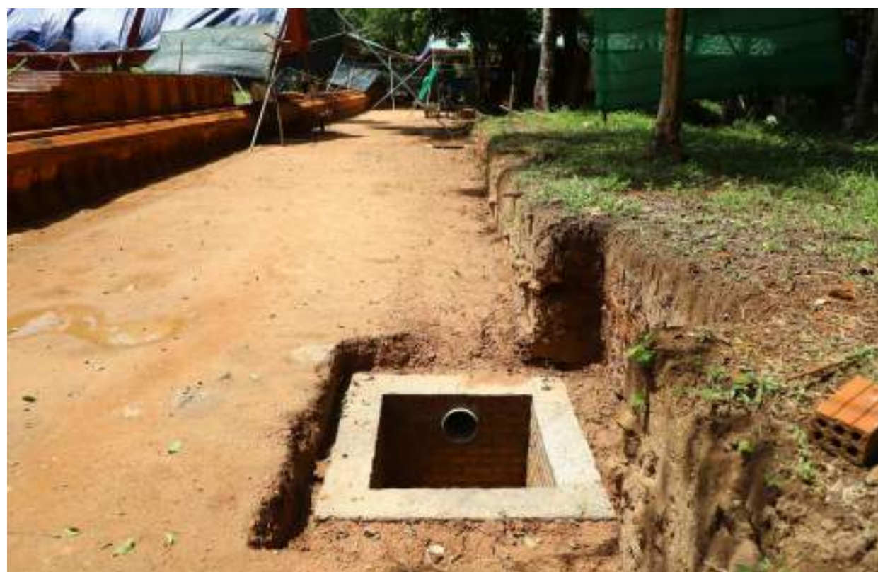
DURING: Construction & Pipe line of Drain Chamber North-west
