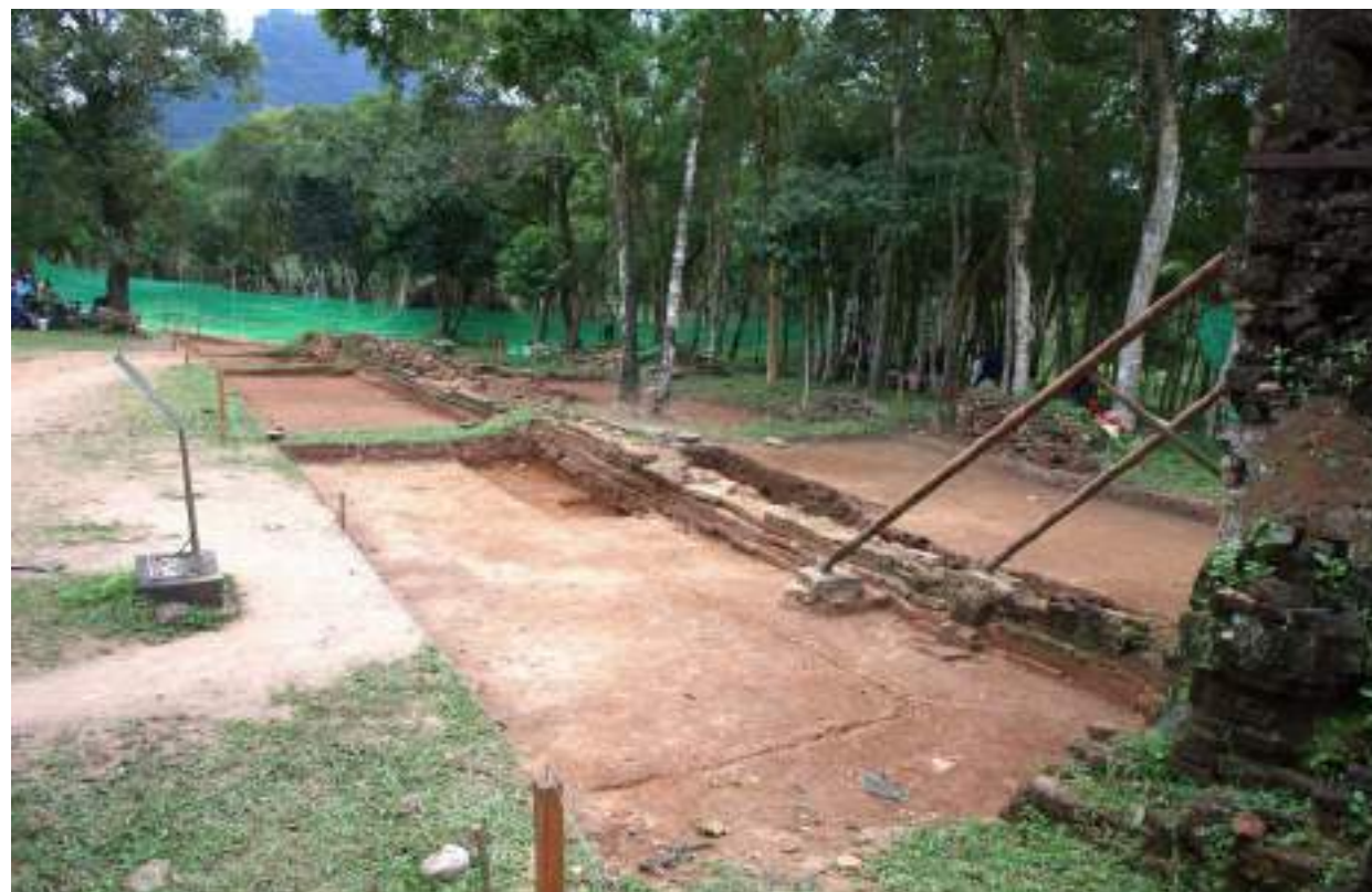
BEFORE: Conservation & Restoration of West Enclosure wall
