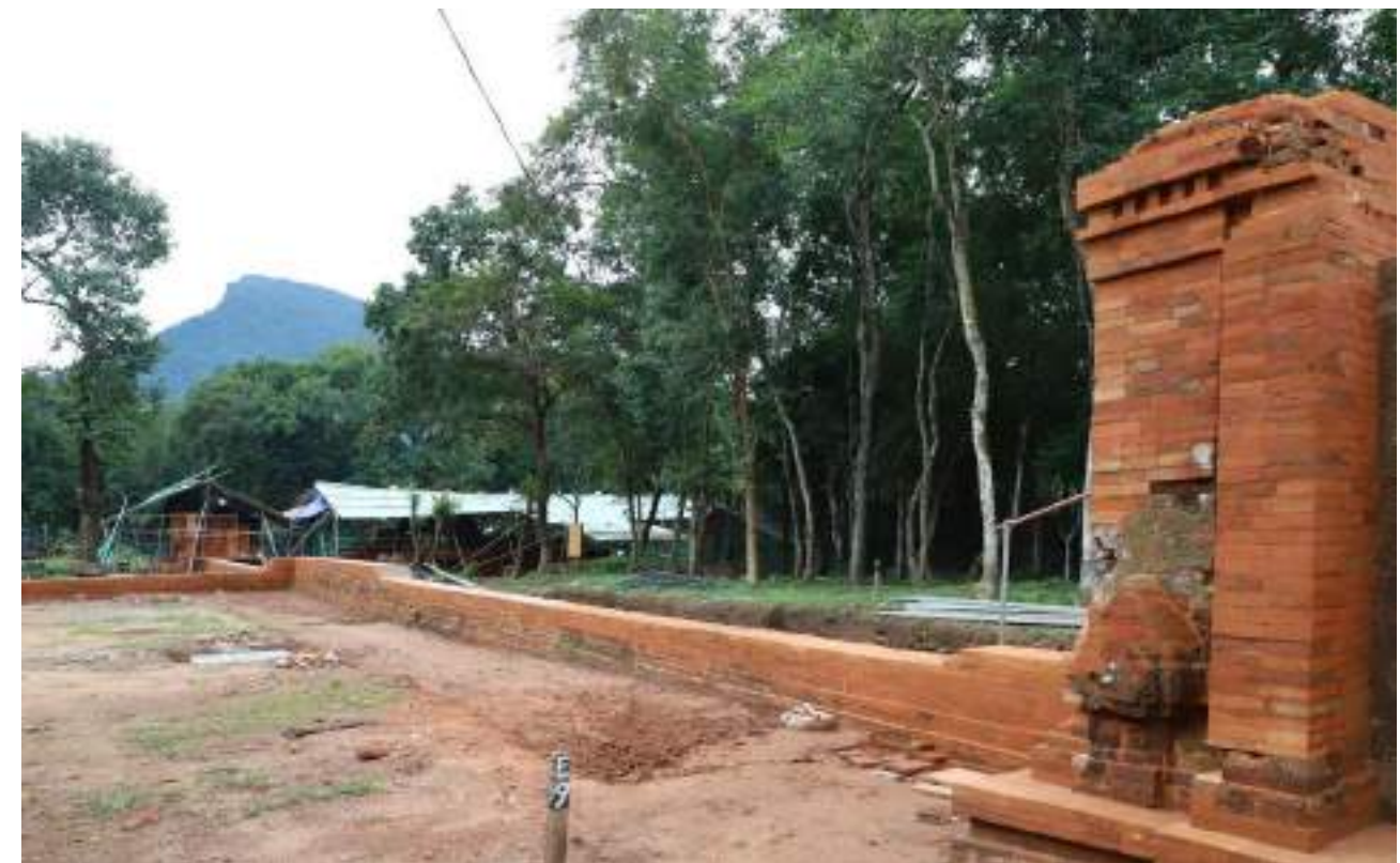
AFTER: Conservation & Restoration of West Enclosure wall
