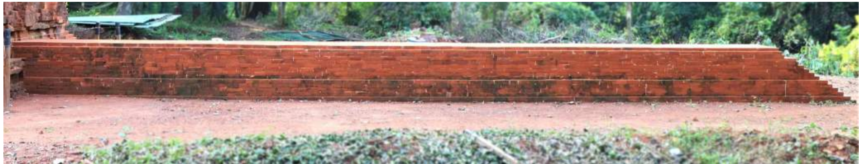
AFTER: Conservation & Restoration of Enclosure wall
