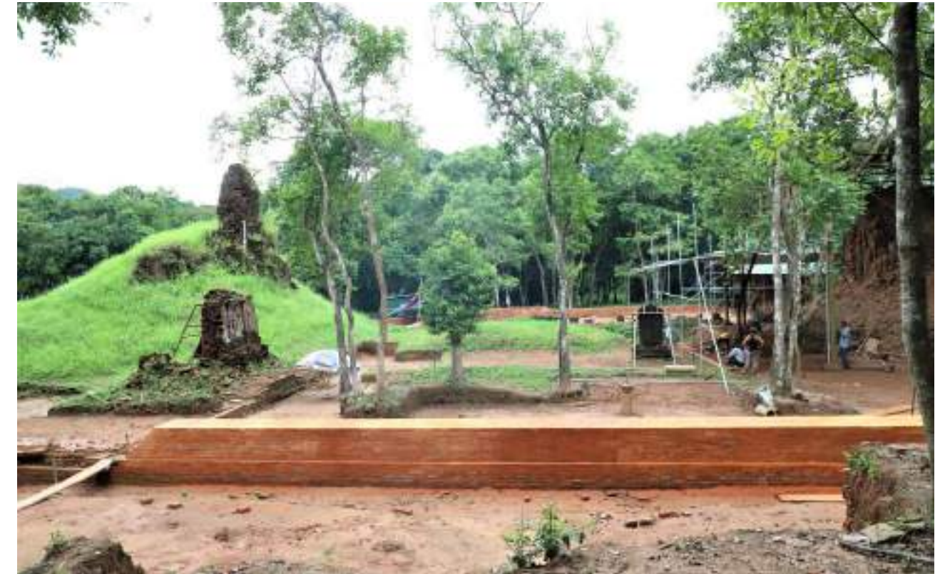
AFTER: Conservation & Restoration of East Enclosure wall
