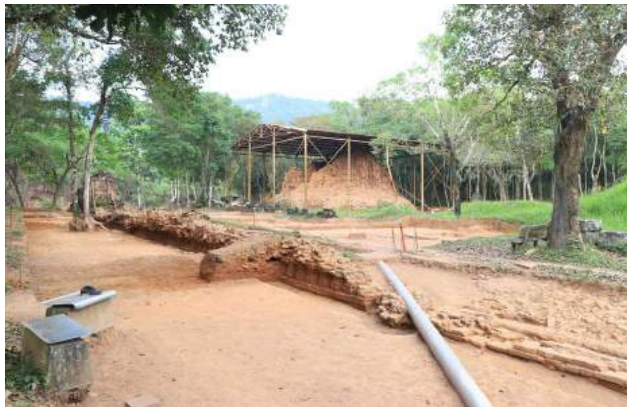
BEFORE: Conservation & Restoration of West Enclosure wall
