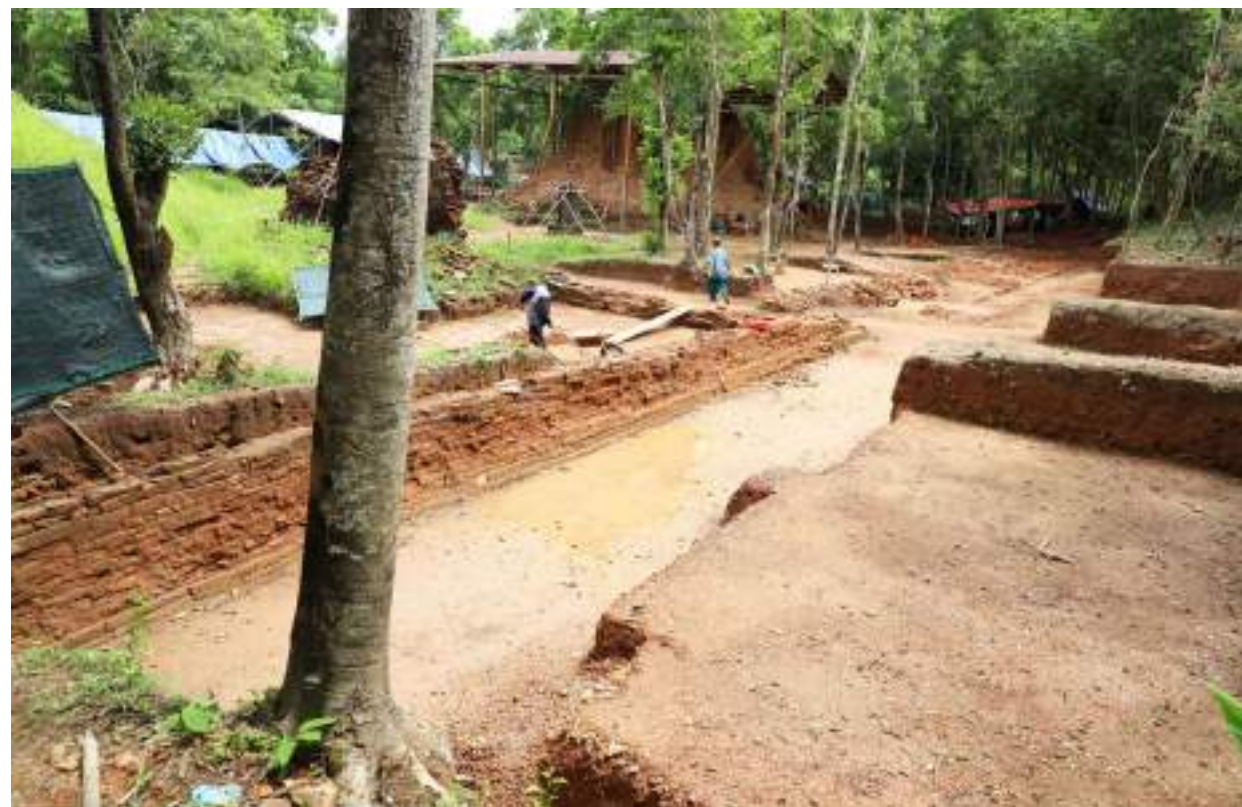
BEFORE: Conservation & Restoration of East Enclosure wall
