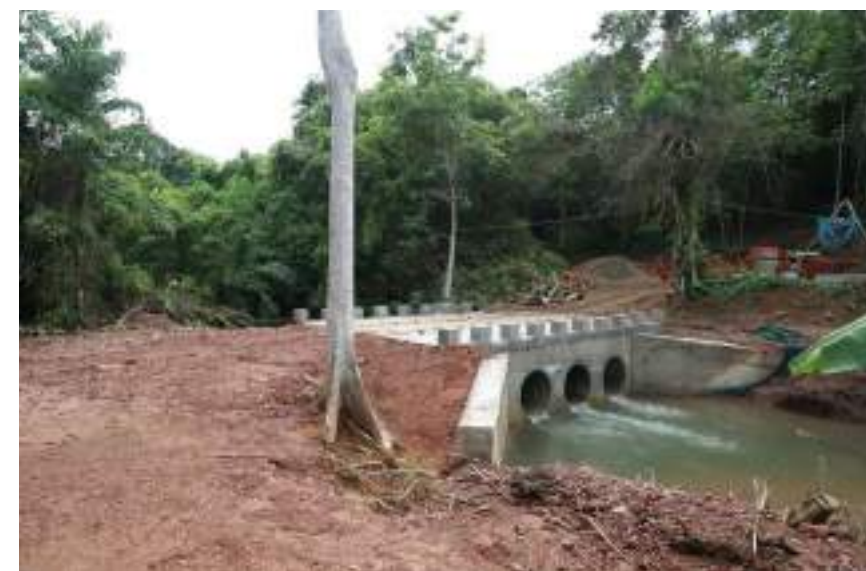
AFTER: Construction of Causeway at Group F temple
