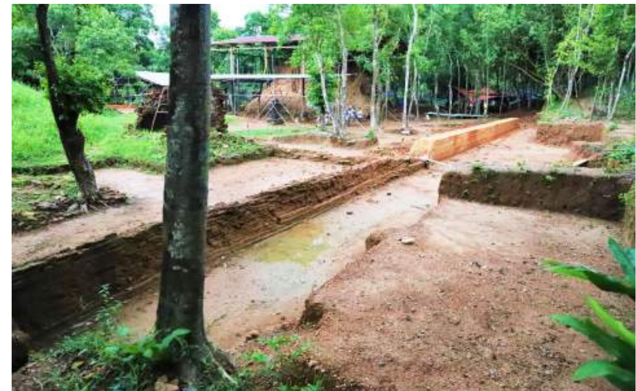
AFTER: Conservation & Restoration of East Enclosure wall
