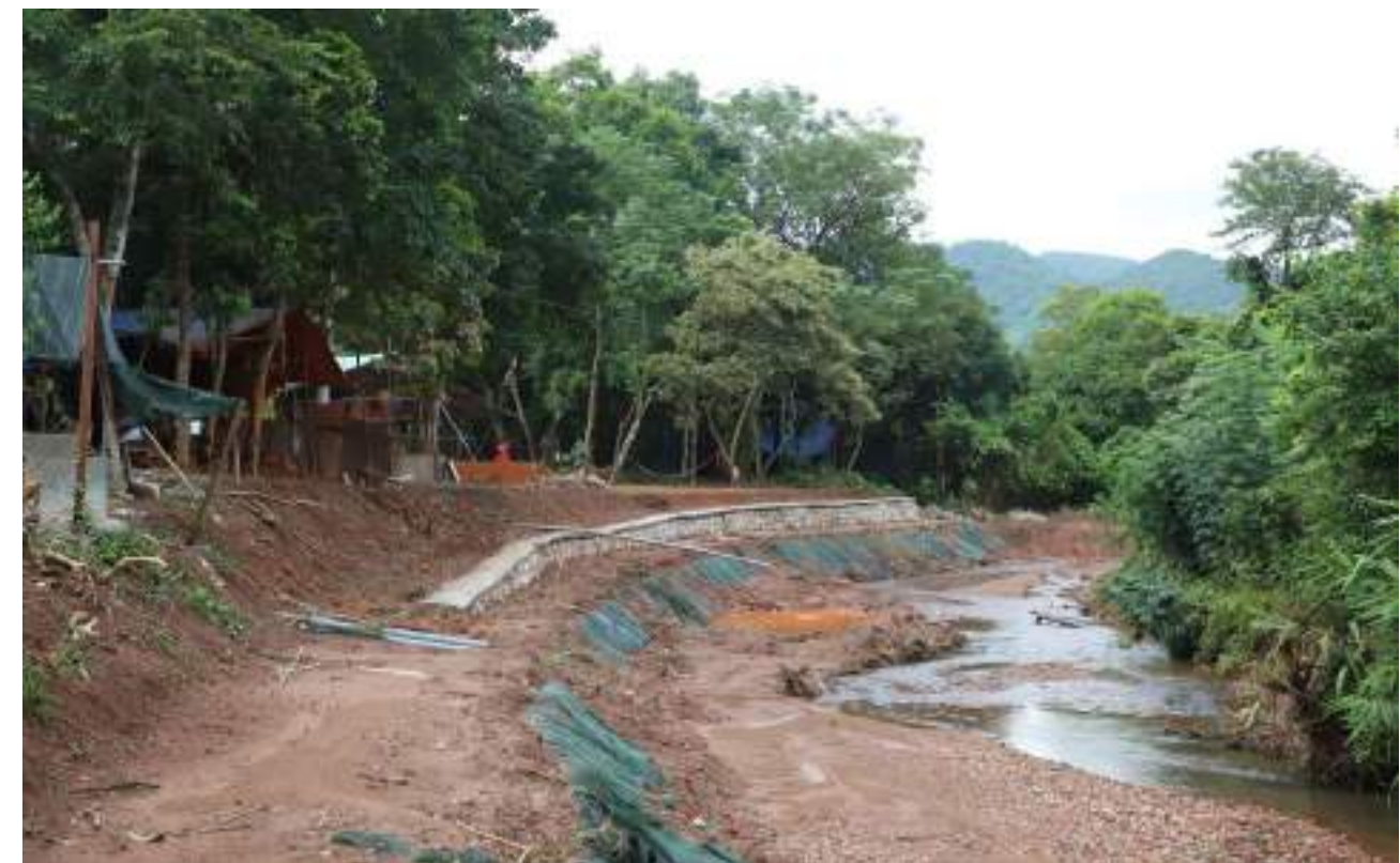
AFTER: East view of Bank protection wall
