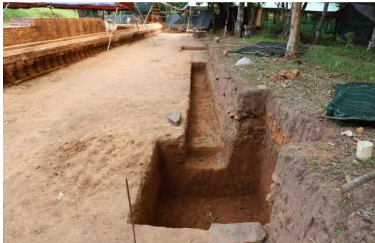
BEFORE: Excavation for Drain Chamber at North-west
