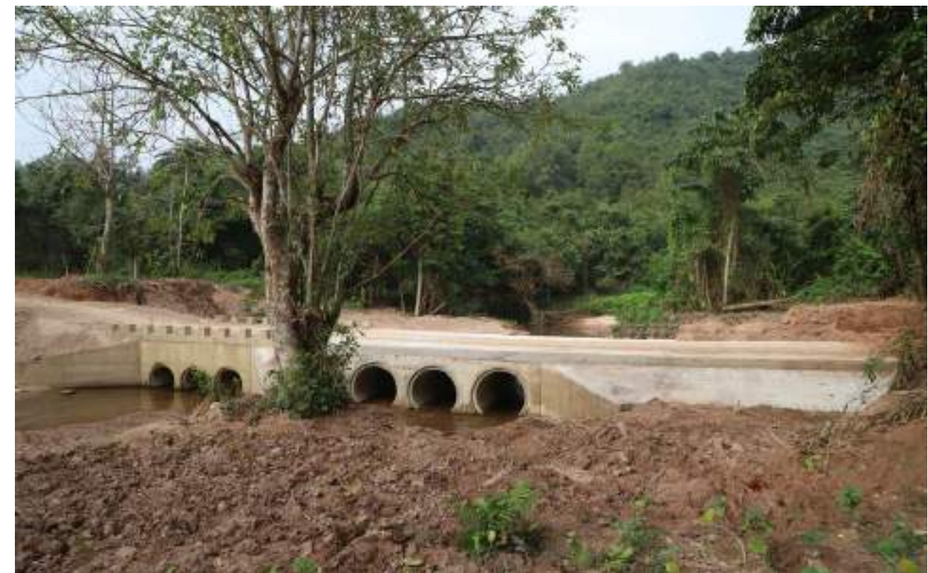
AFTER : Construction of Causeway at Group K
