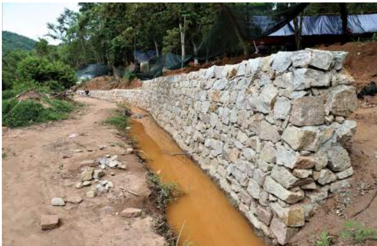
DURING: Construction of Bank protection wall
