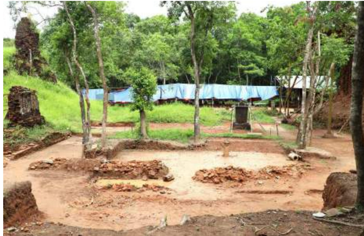
BEFORE: Conservation & Restoration of East Enclosure wall
