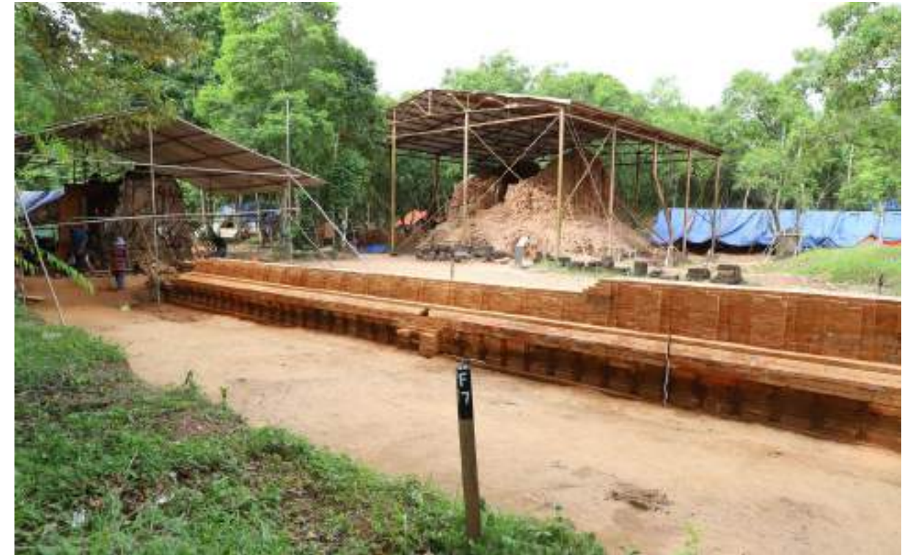
AFTER: Conservation & Restoration of West Enclosure wall
