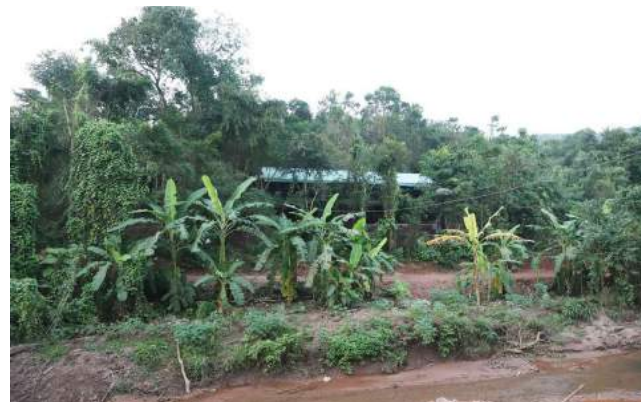
Erected Worker Shed
