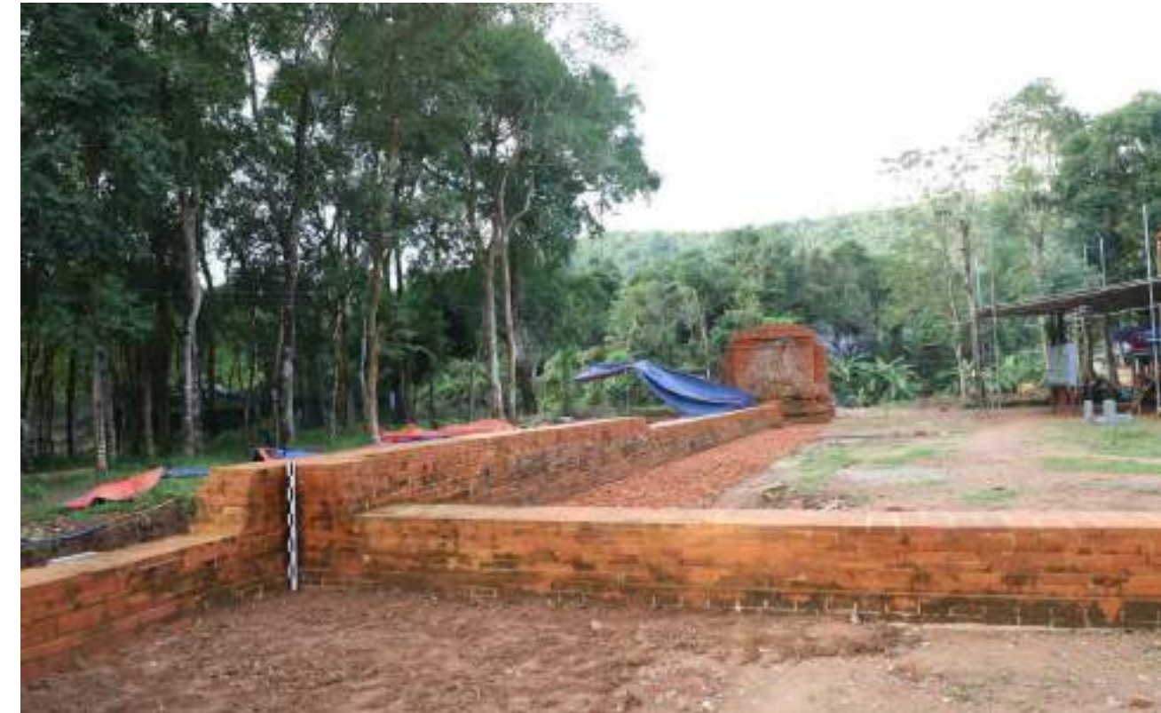
AFTER: Conservation & Restoration of West Enclosure wall
