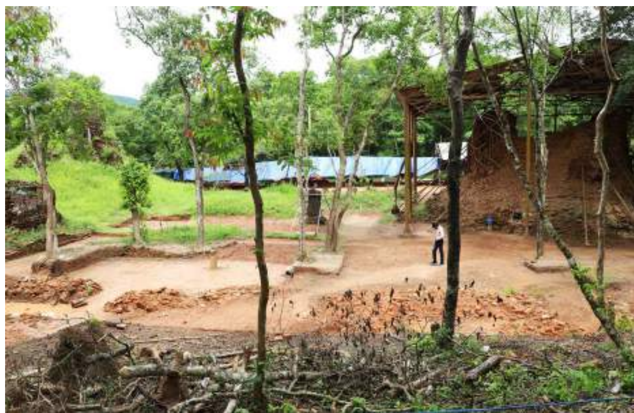
BEFORE: Conservation & Restoration of East Enclosure wall
