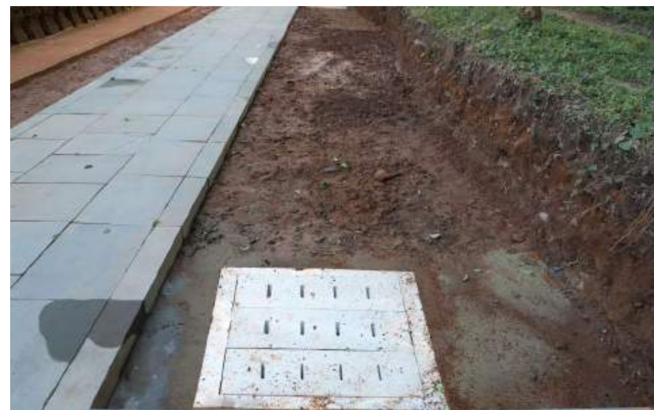
AFTER: Construction of Drain Chamber North-west
