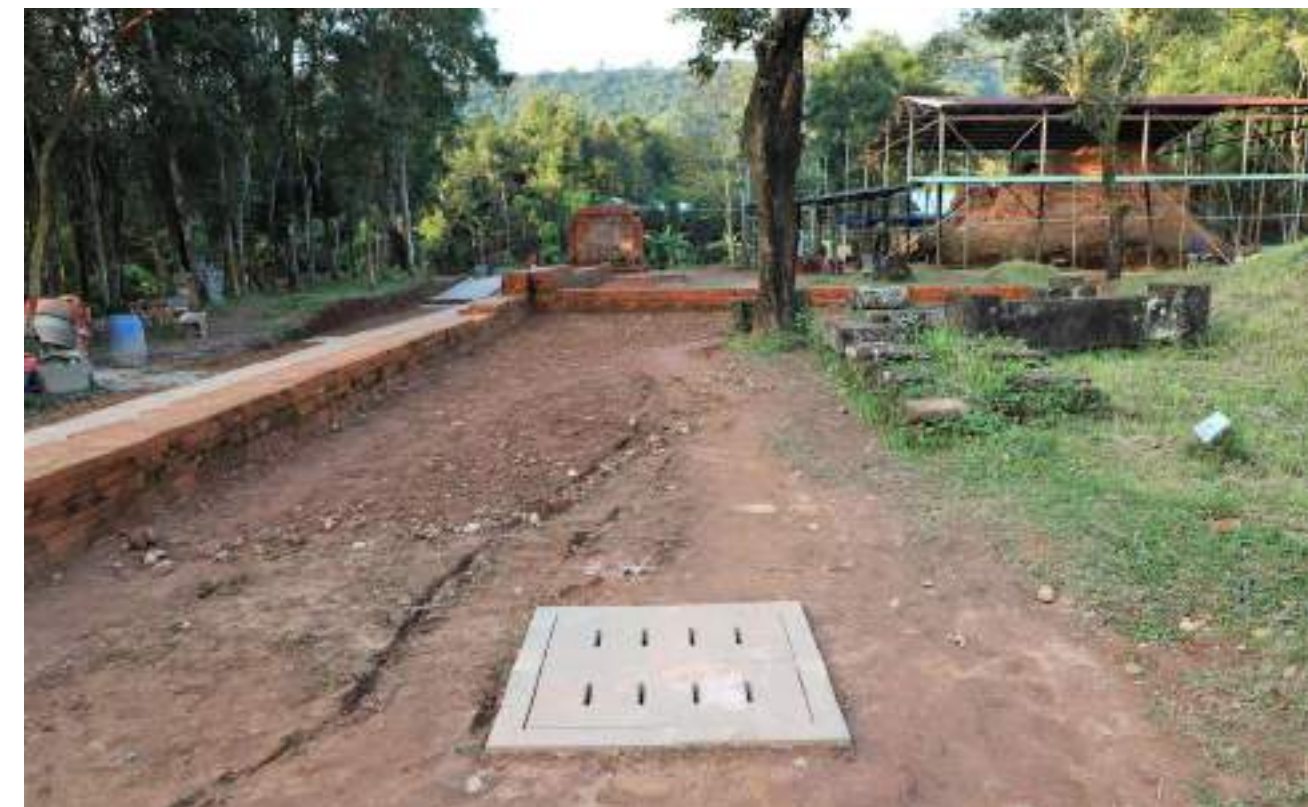
AFTER: Construction of Drain Chamber at south east
