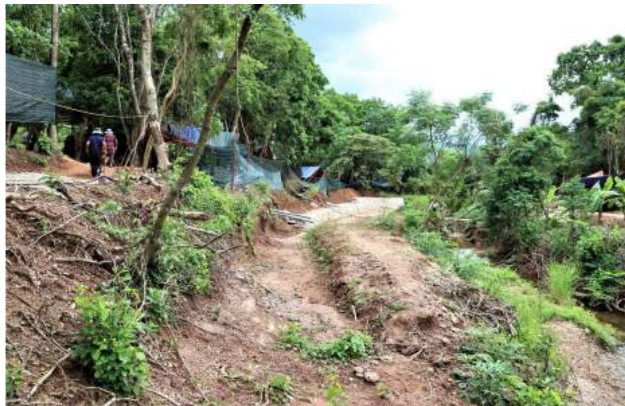
DURING: Construction bank protection wall
