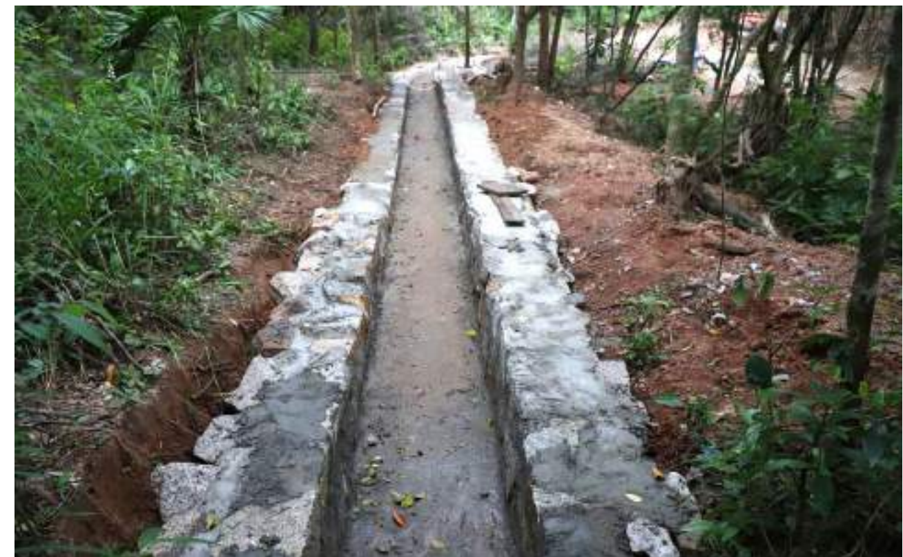
AFTER: Construction of Contour Drain
