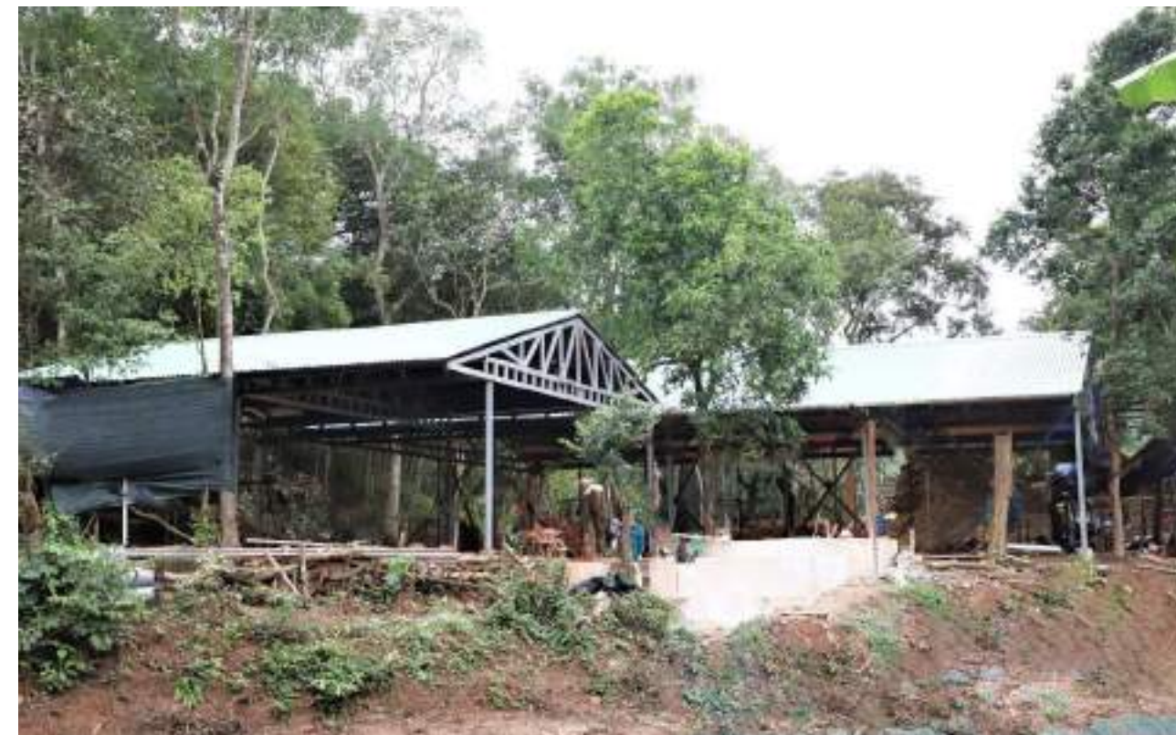
Erected Working Shed
