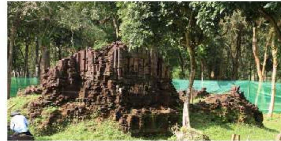
E-Group Before: Condition of structure
