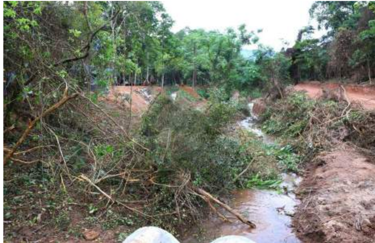
BEFORE: Bank protection wall
