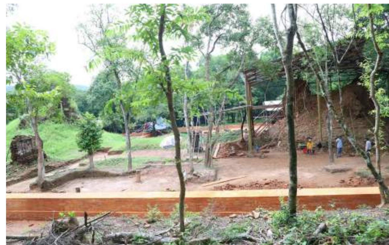
AFTER: Conservation & Restoration of East Enclosure wall
