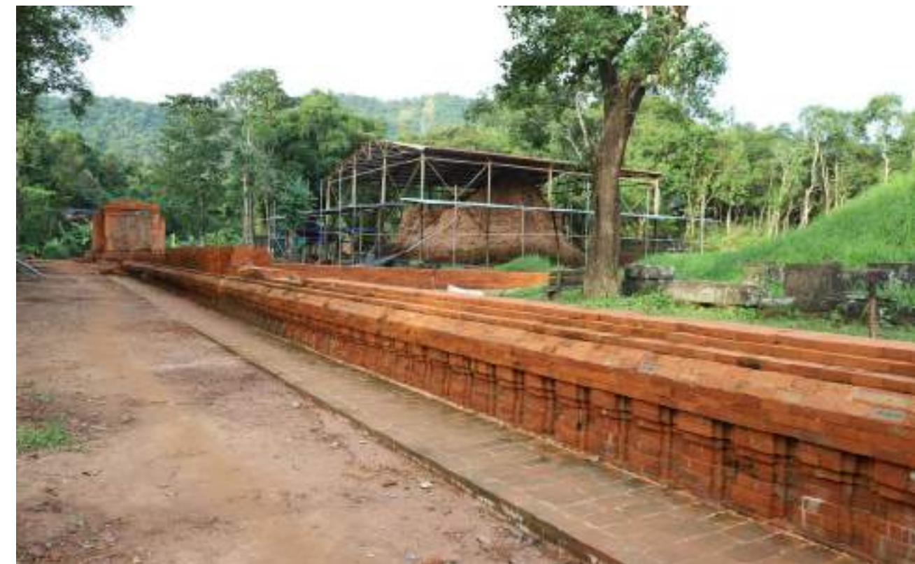
AFTER: Conservation & Restoration of West Enclosure wall
