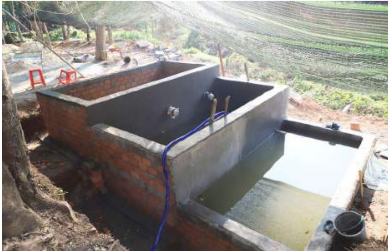
Construction of Lime Slacking tank
