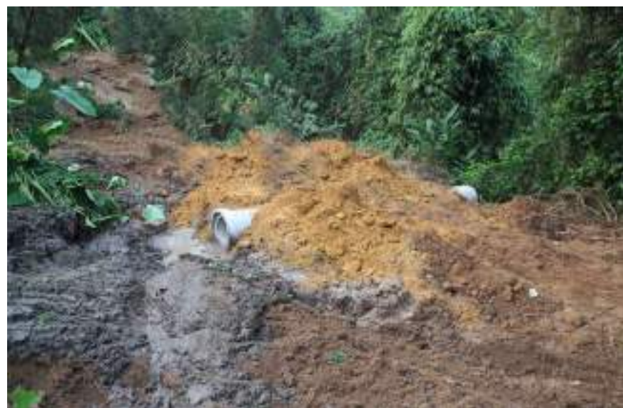
BEFORE: Construction of Causeway at Cham Hut
