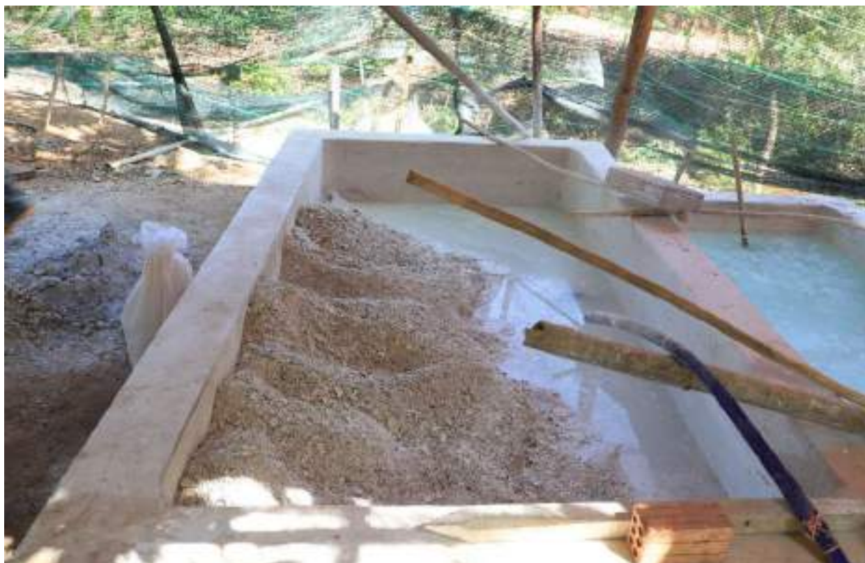
Lime Slacking Process
