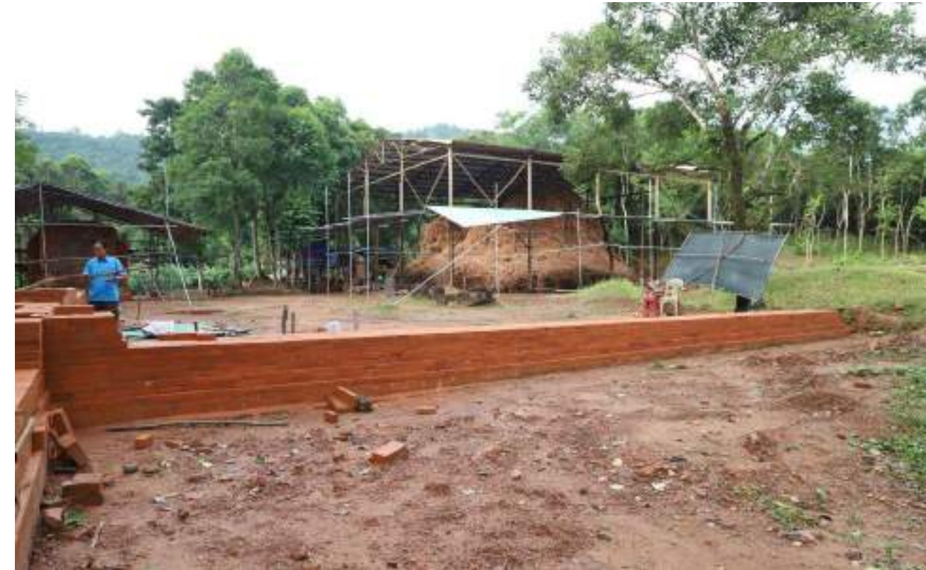
AFTER: Conservation & Restoration of partition Enclosure wall
