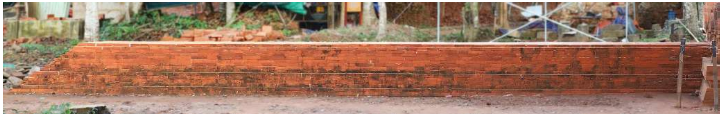
AFTER: Conservation & Restoration of Enclosure wall
