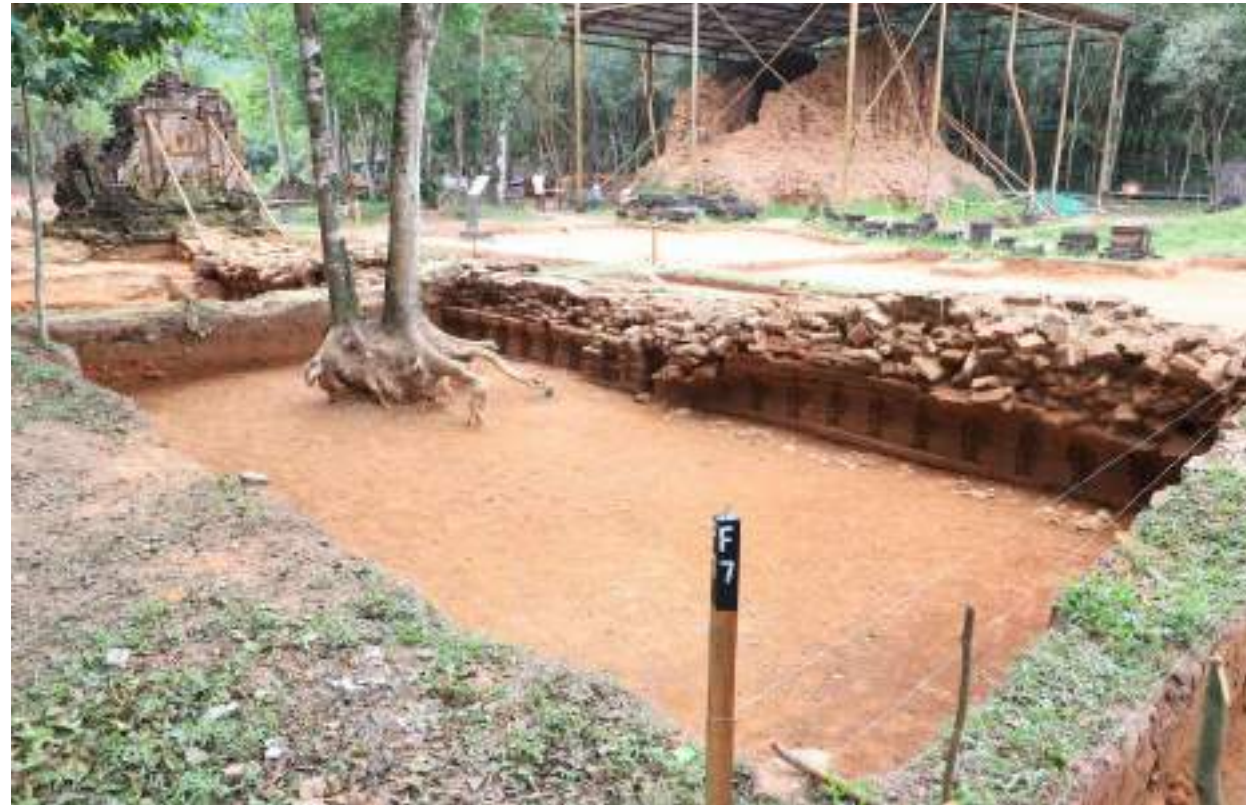
BEFORE: Conservation & Restoration of West Enclosure wall
