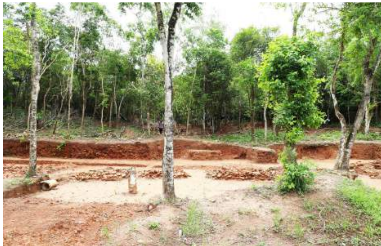
BEFORE: Conservation & Restoration of East Enclosure wall
