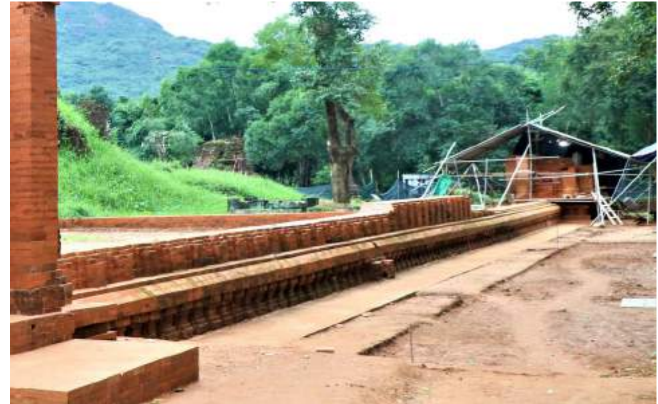
AFTER: Conservation & Restoration of West Enclosure wall
