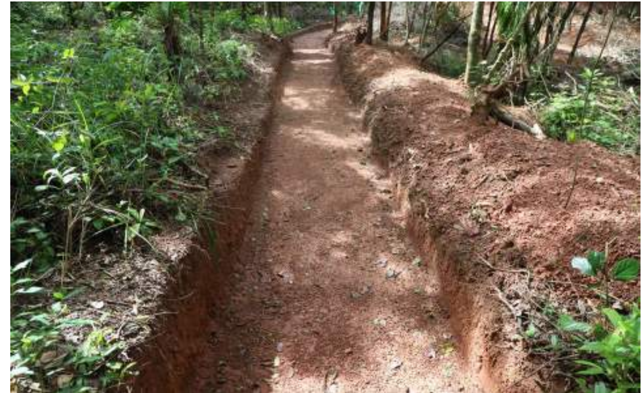
DURING: Excavated area for Contour Drain
