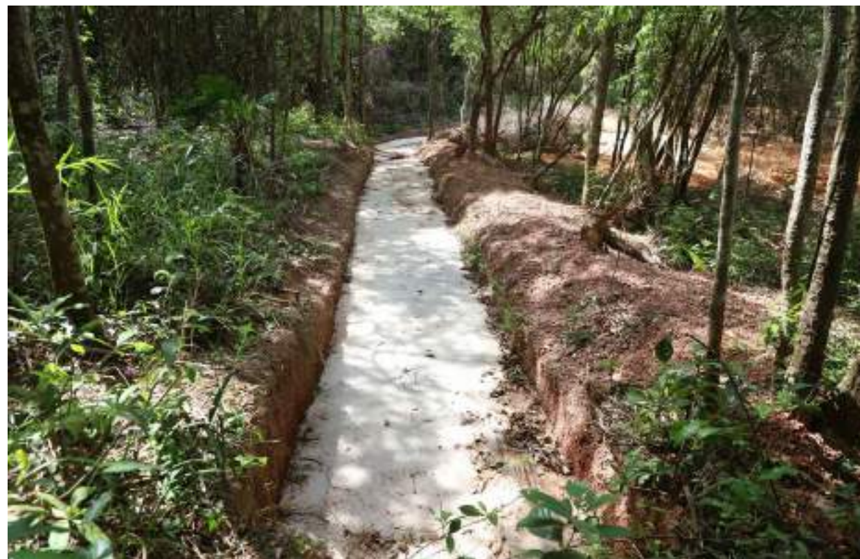
DURING: Laying of PCC for Contour Drain
