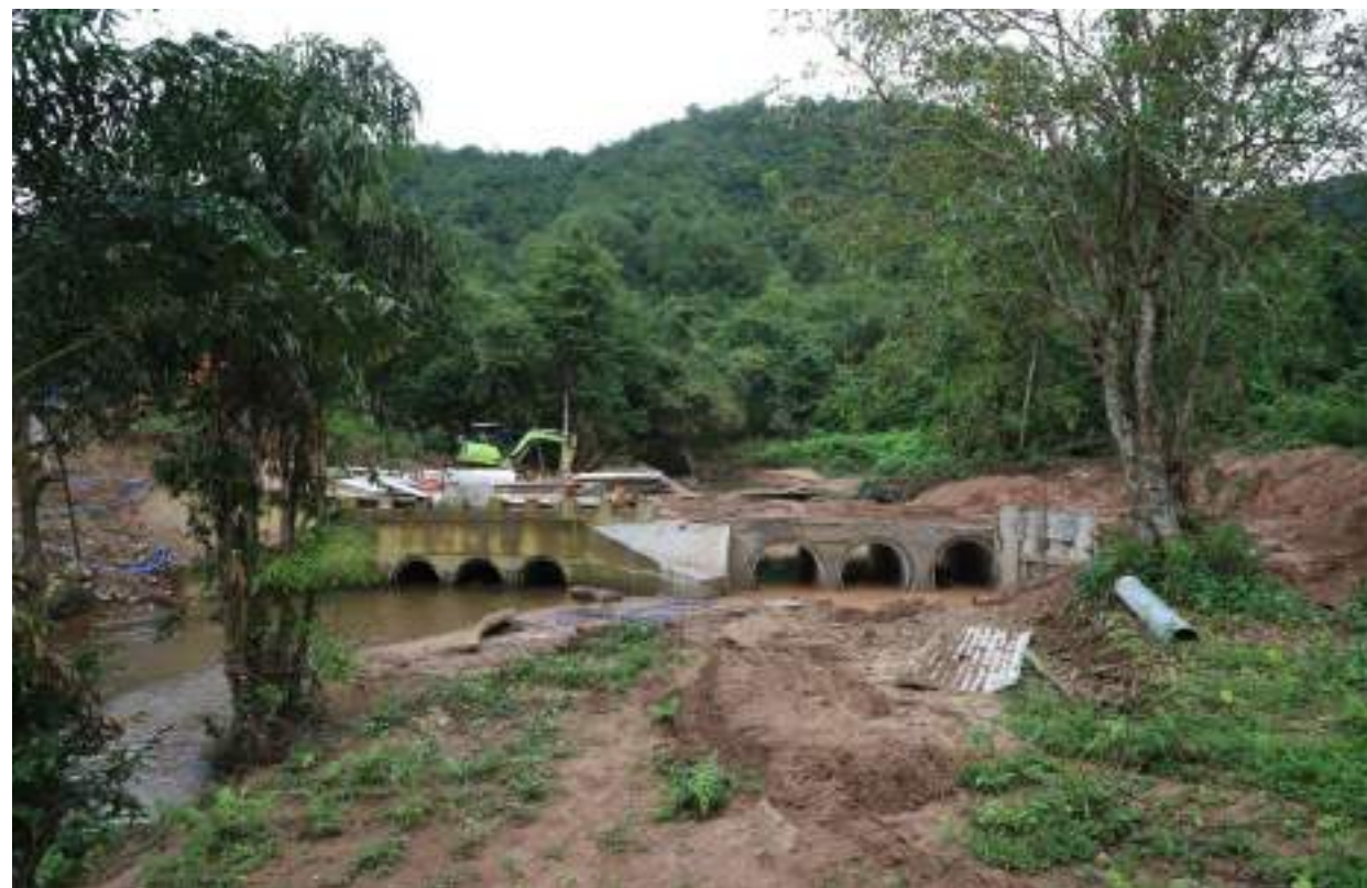
DURING : Construction of Causeway at Group K
