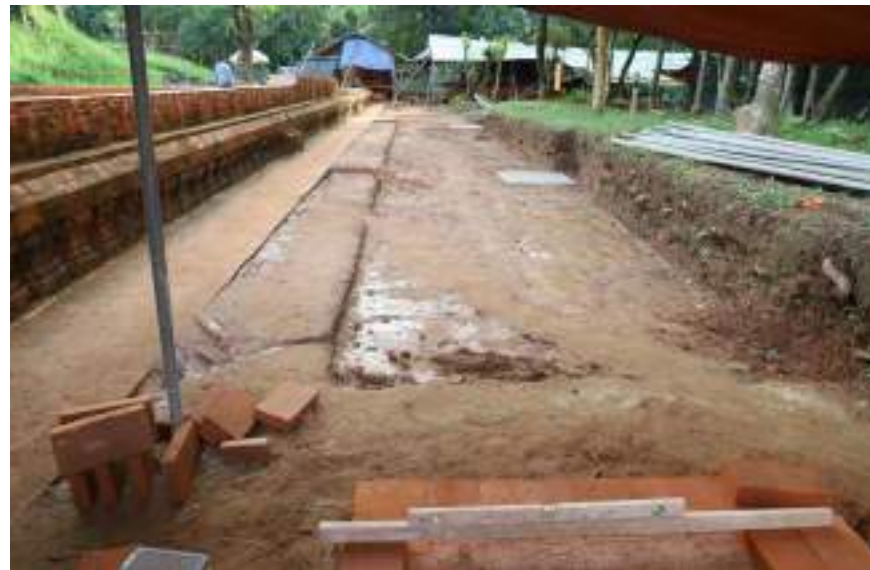
BEFORE: Pathway from north to south
