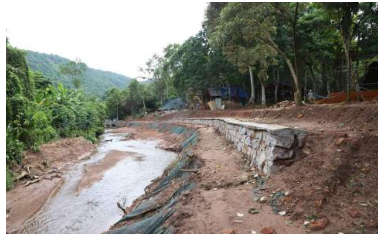
AFTER: West view of Bank protection wall
