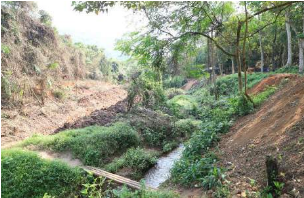
BEFORE: Bank protection wall
