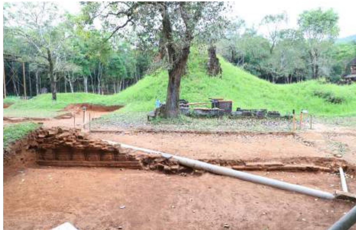
BEFORE: Conservation & Restoration of West Enclosure wall
