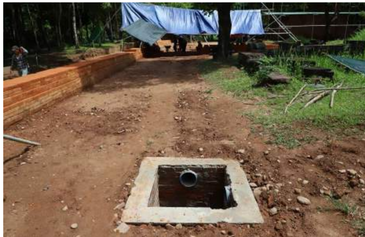
DURING: Construction & Pipe line of Drain Chamber at south east
