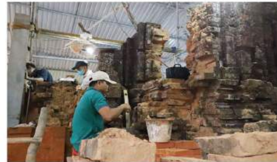
E-Group During: Numbering, dismantling & restoration
