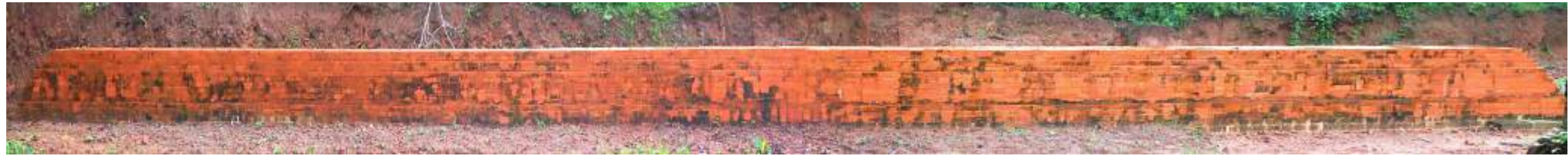
AFTER: Conservation & Restoration of Enclosure wall
