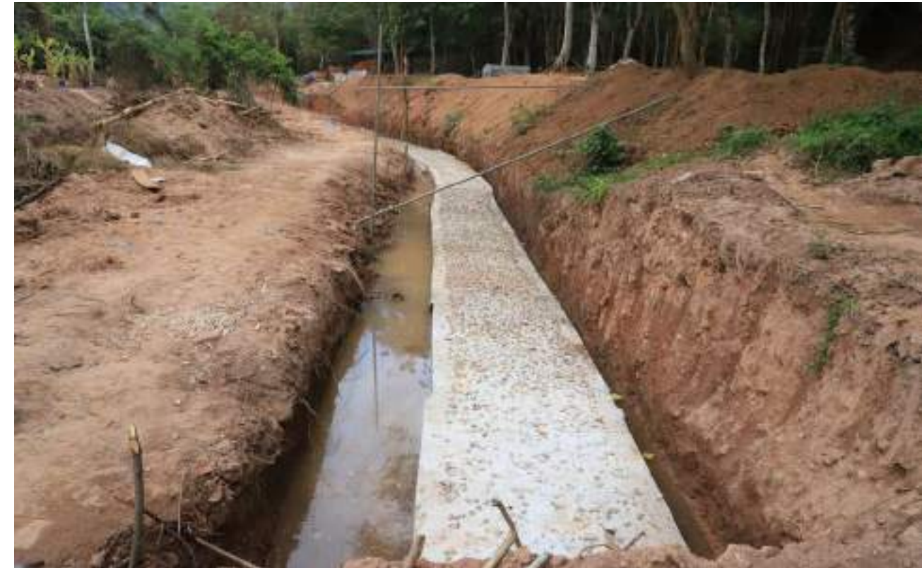
DURING: Construction of Bank protection wall
