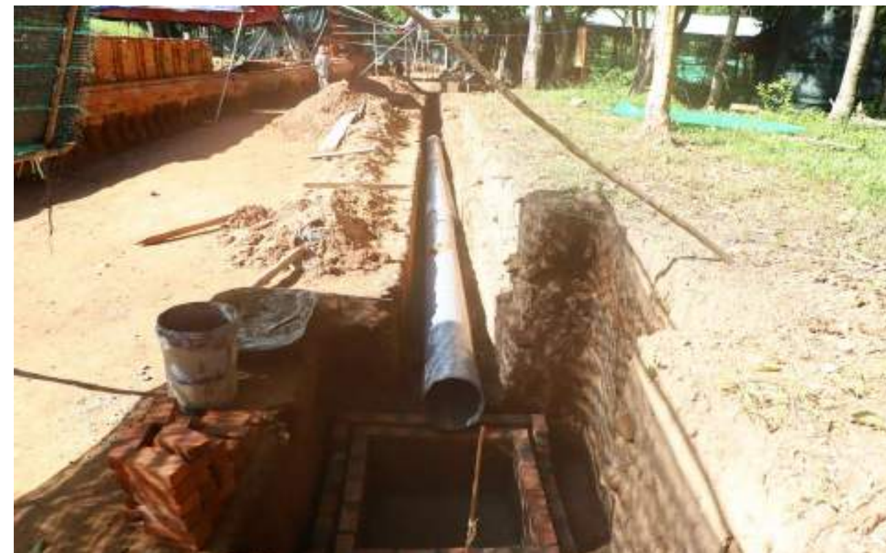
DURING: Construction of Drain Chamber North-west
