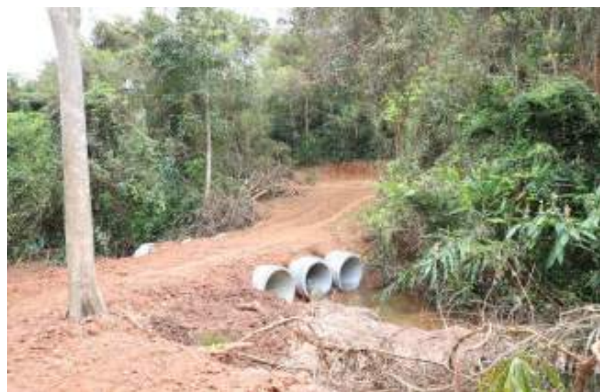
BEFORE: Construction of Causeway at Group F temple
