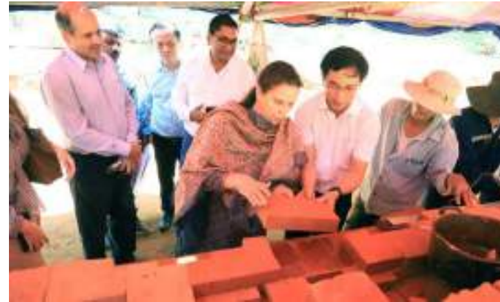
Sri Sandeep Arya, H E Ambassador of India to Socialist Republic of Vietnam inspection of Ongoing activity at the site
