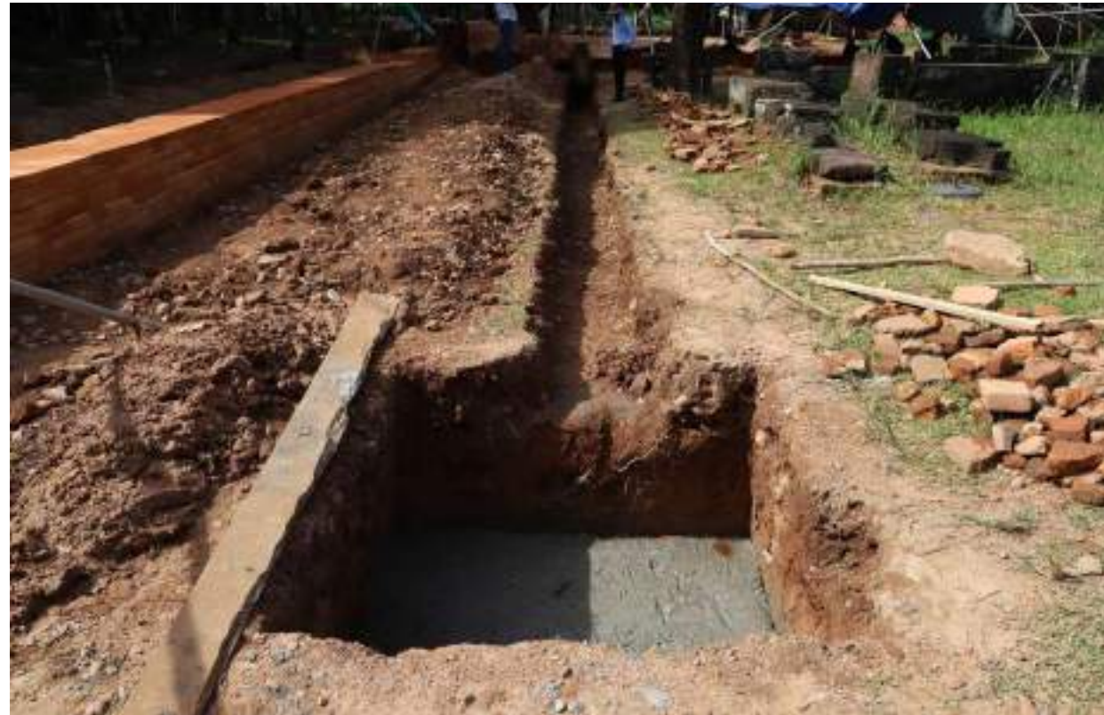
BEFORE: Excavation for Drain Chamber at south east
