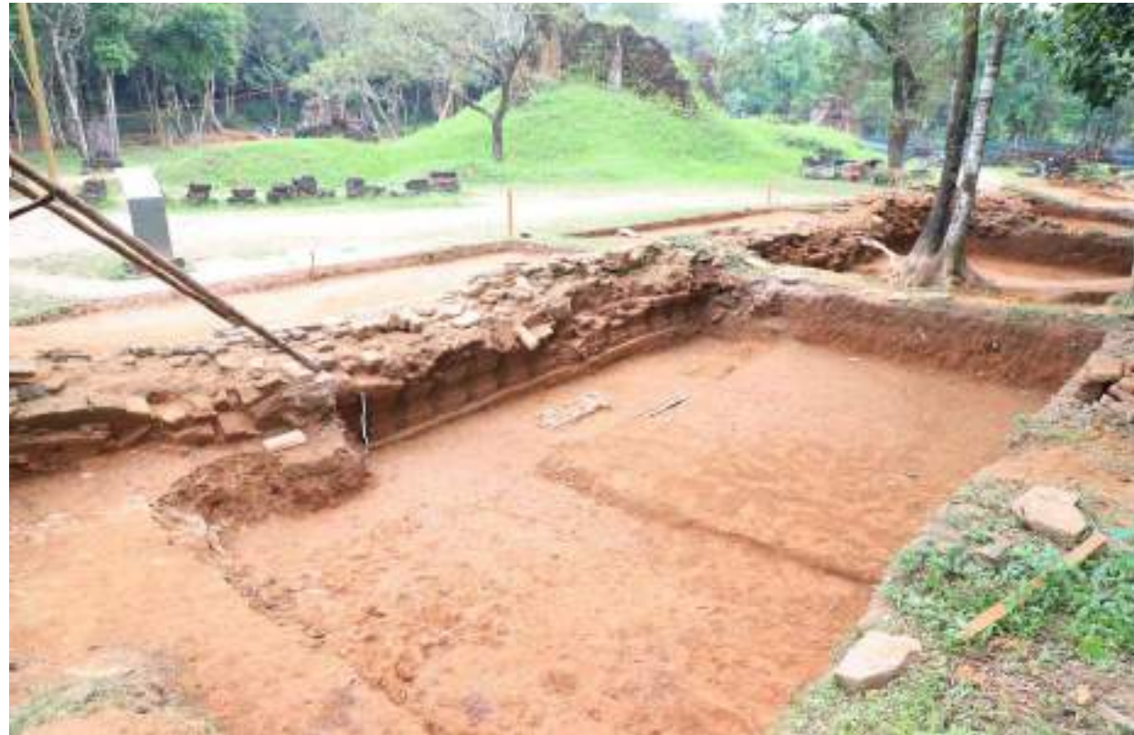
BEFORE: Conservation & Restoration of West Enclosure wall
