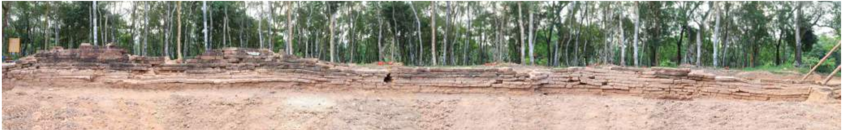
BEFORE: Conservation & Restoration of West Enclosure wall
