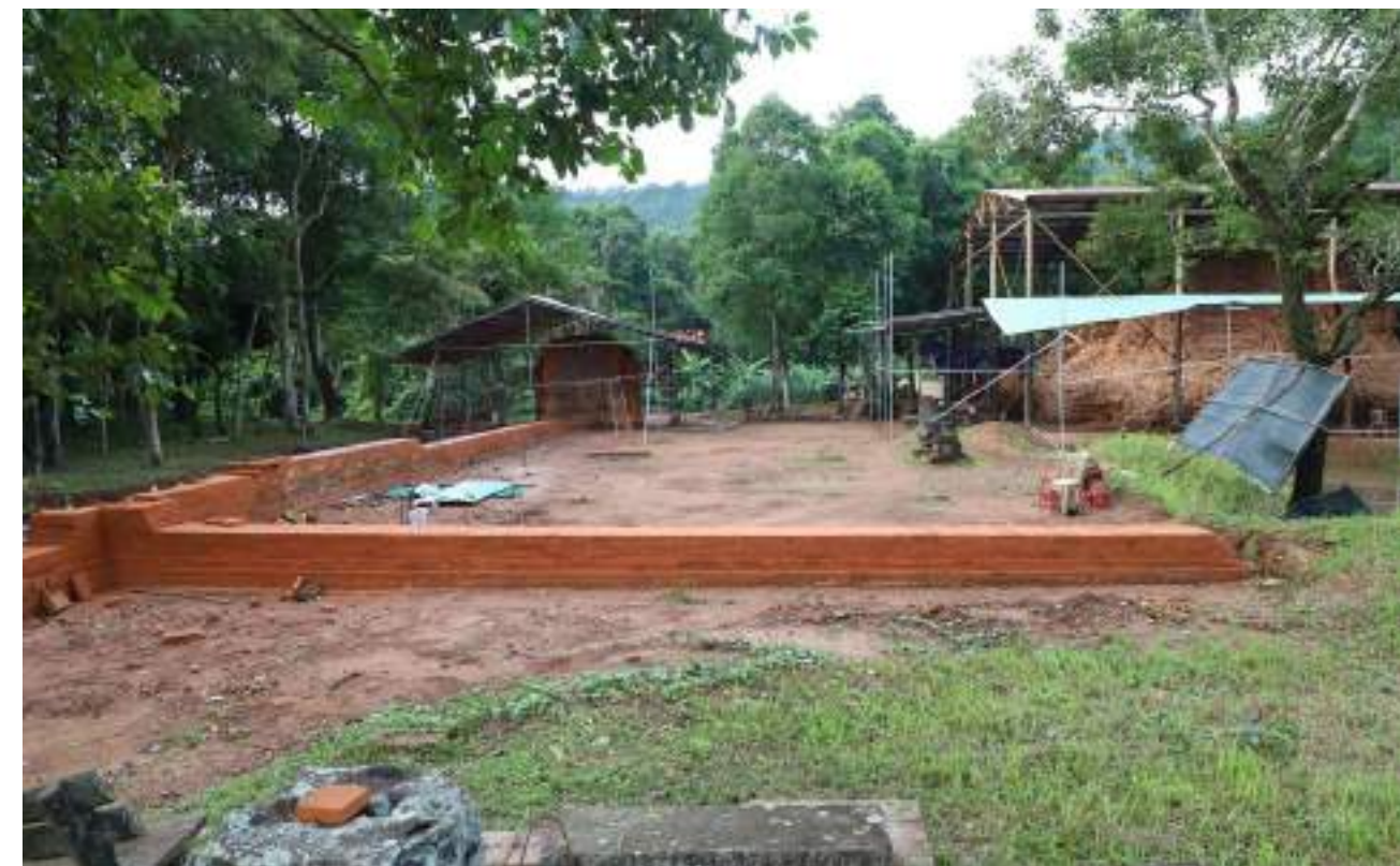
AFTER: Conservation & Restoration of partition Enclosure wall
