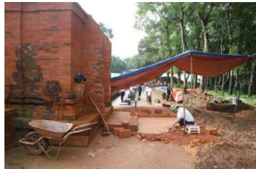
BEFORE: Pathway from north to south
