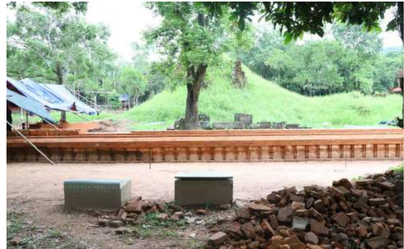
AFTER: Conservation & Restoration of West Enclosure wall
