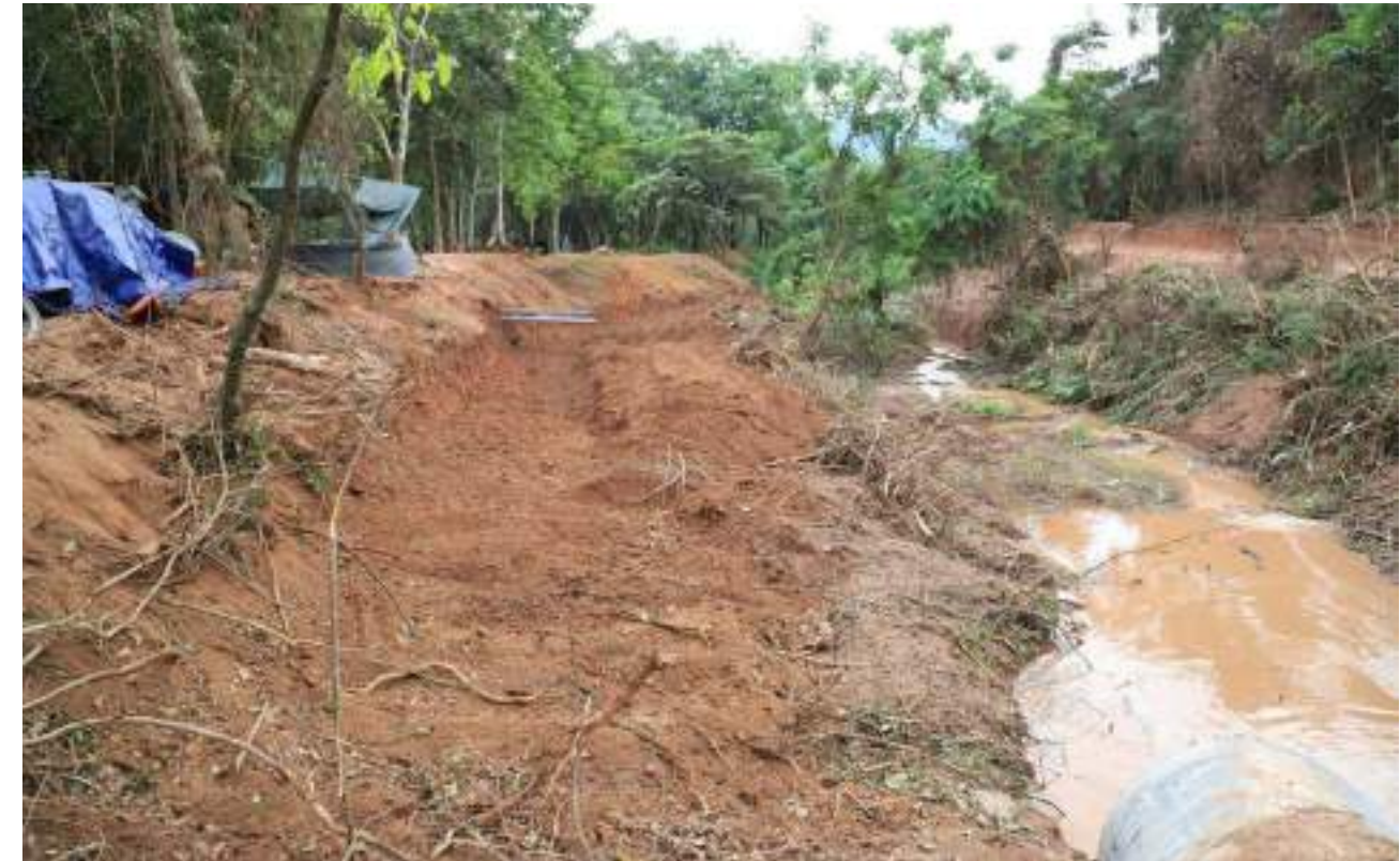
DURING: Construction bank protection wall
